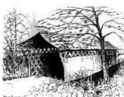
Eastley Bridge Blount County, AL
